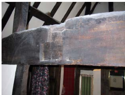
Mortice in tie beam
